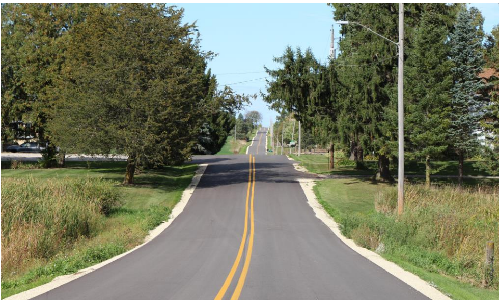
The segment of demonstrates a PASER rating of “9” (2023) due to newly installed asphalt surface.
